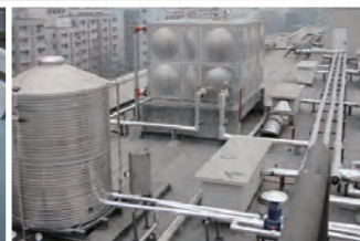
Water tank fabrication
